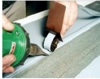
- Junction seals weld -
